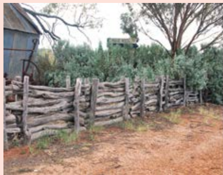
The fence was built from a local timber (eucalyptus), which is a common sight in the region, and was made of square posts and round rails.
